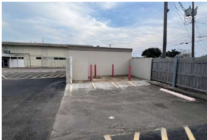
Enclosed dumpster area
