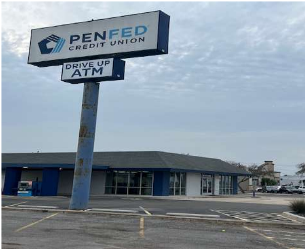
View of Pole Sign and Building from Staples St.
