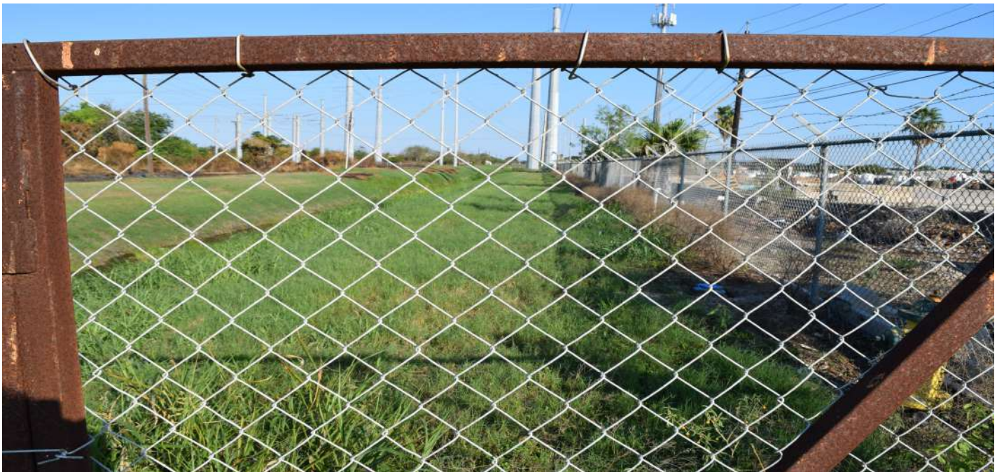
Gate which leads to access to La Costa Dr. at rear of property
