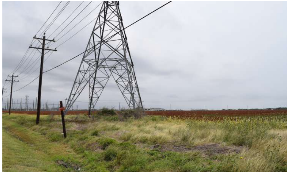
NW corner of property looking south on CR 69 with transmission line visible
